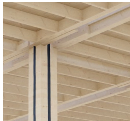
Mustermaja laesõlm The Pattern Building ceiling joint
