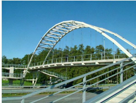
E20, pedestrian bridge
